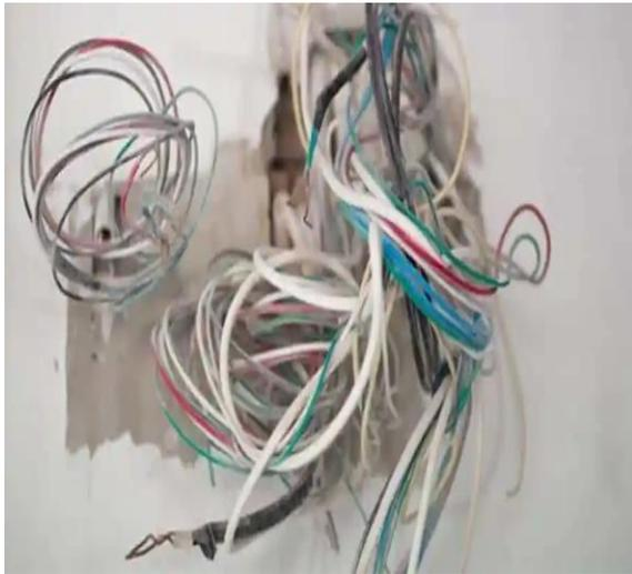
*Fig. 7: Overcrowded Electrical Wiring*
