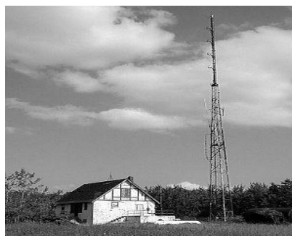
A Typical Rural Radio Network Transmitter Site
