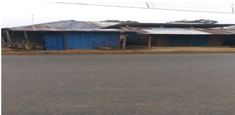
Figure 4: Temporary Structures/Containers in the Study Area located too close to the Road
