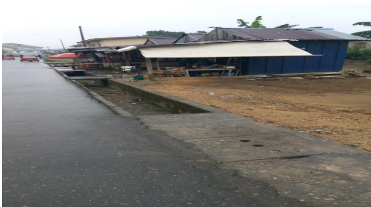
Figure 6: Temporary Structures/Containers located in close proximity to each other
