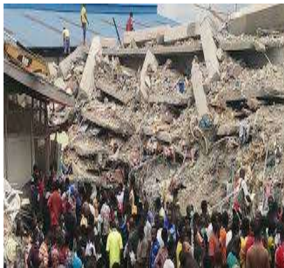
Fig. 2: The Synagogue Church of All Nations (SCOAN) Guesthouse Collapse
