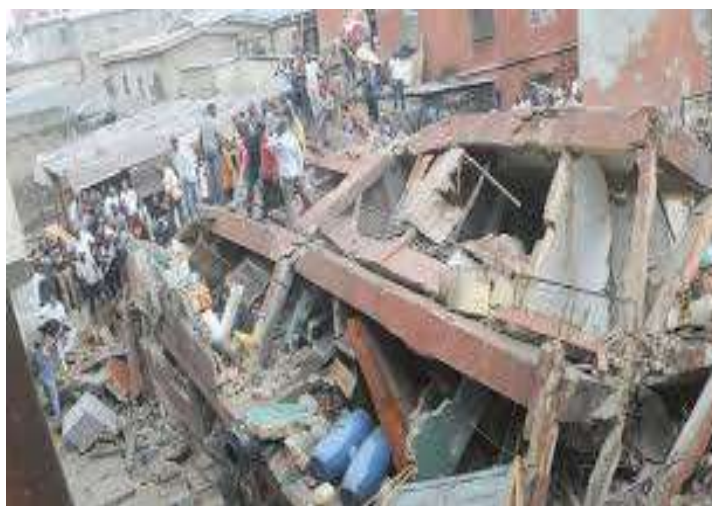
Fig. 4: Ita-Faaji School Building Collapse
