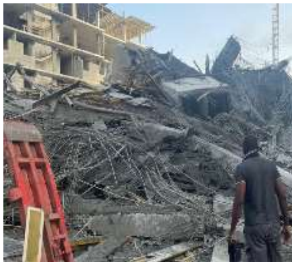
Fig. 8: Collapse of a two-story Saint Academy school building in Jos
