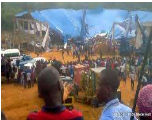
Fig 1. Building collapse scene.
