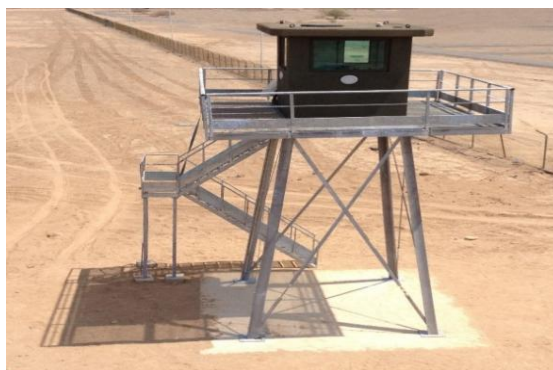
Fig. 6: Mobile Observation Towers
